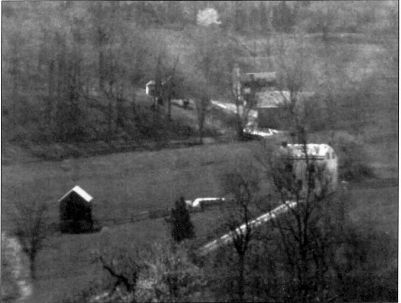
This previously unpublished photograph, taken in 1909 by W.R. Jennings, is the first known image of the Church Road Cabin, and looks south across the Great Valley from a vantage point on the North Mountain. Church Road runs diagonally across the foreground of the image. Beyond Valley Creek, which runs horizontally across the photograph, can be seen the two-story log structure, with its spring house on the left, and two mill-related structures on the right side of Church Road, all owned at that time by the estate of George Fetter. Courtesy of St. Peter's Church in the Great Valley.
