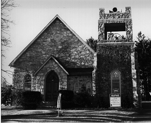
Figure 3. Nottingham Presbyterian Church, constructed of serpentine from the Dunlap and Martin quarry in Nottingham County Park.
