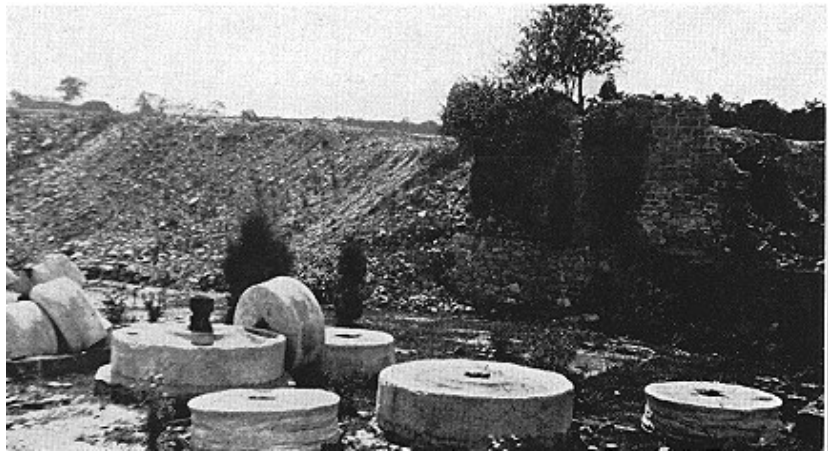
Figure 25. Burrstones, waste piles, and ruins of a mill at the Sparvetta Mining Company, south of NCP, where part of the output from the Brandywine Quarry was ground. (Stone and Hughes, 1931, Plate III)
