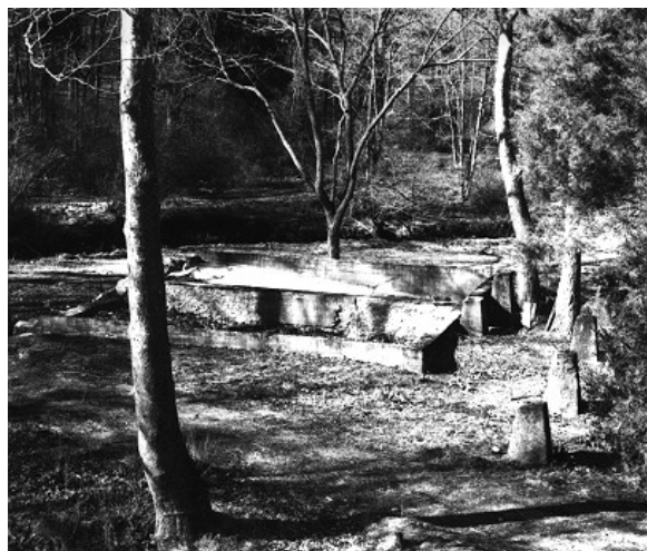
Figure 20. Concrete foundation piers of a mill constructed in NCP during World War I for the recovery of placer chromite.
