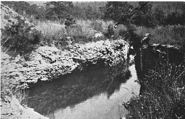
Figure 26. Feldspar pit in NCP described as “near Cooper log house in The Barrens, showing swell and pinch of the dike.” (Stone and Hughes, 1931, Plate IV) (Close examination will reveal what appears to be a meteorite about to make impact. This image appeared in all copies of Stone and Hughes’ report. Is it purely coincidental that, one year after the publication of this report, Ralph Stone teamed up with Eileen Starr to publish Meteorites Found in Pennsylvania? )
